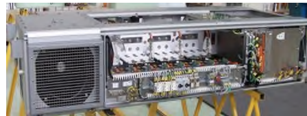
Main IGBT converter. Dual voltage 600/1500 Vdc
